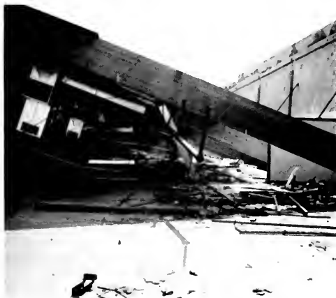
Photo 17. Collapsed roof, Bradley light industrial tract.
